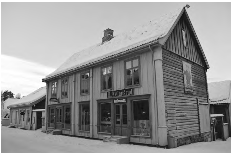
Obr. 2. Avlangrudov obchod so zmiešaným tovarom, expozičný celok Mesto, Maihaugen, Stiftelsen Lillehammer museum v Lillehammeri. Foto R. Sýkora, 2017 Fig. 2. Avlangrud's grocery shop, Urban exhibition unit, Maihaugen, Stiftelsen Lillehammer museum in Lillehammer. Photograph by R. Sýkora, 2017
